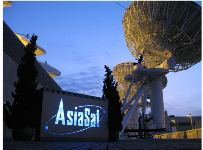
AsiaSat’s state-of-the-art earth station in Hong Kong.
